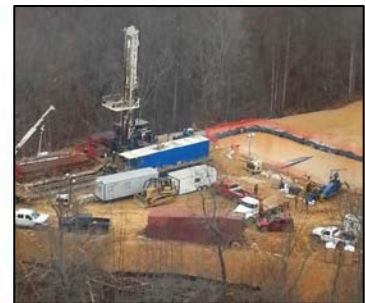
Horizontal Berea Oil Drilling Rig Operations
